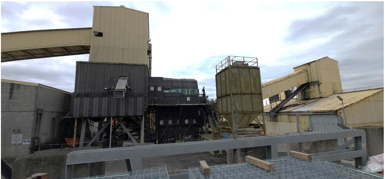
Plate 10 Coal handling plant
