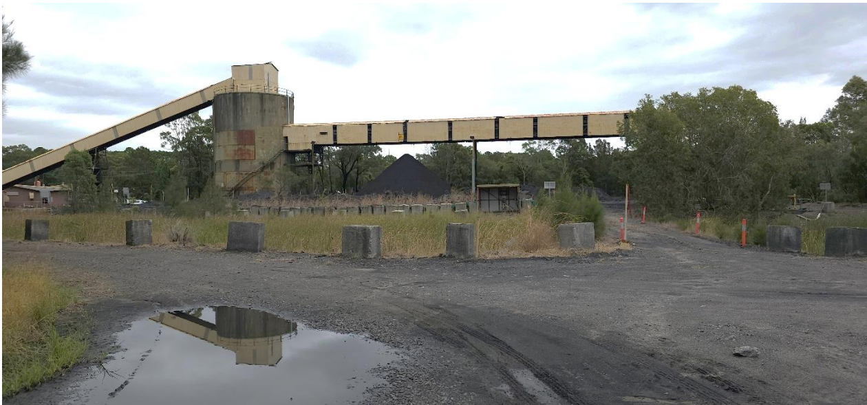
Plate Coal bin and coal stockpile area
