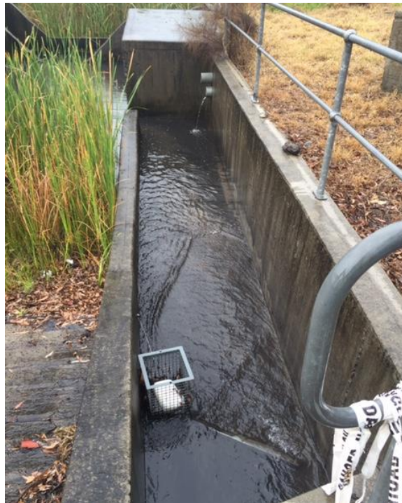
Photo 1. Flocculent block located adjacent the coal stockpile area.
